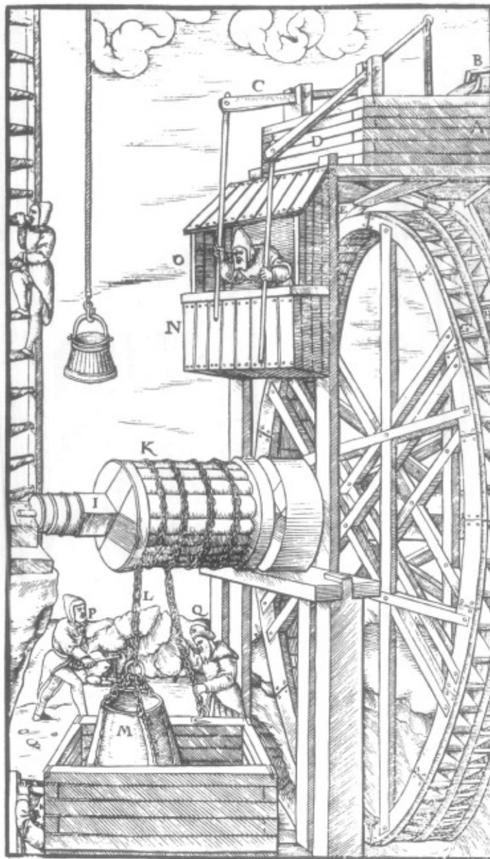
*A wooden water-wheel helps these workmen to remove water from a mine. (Burndy Library)*
