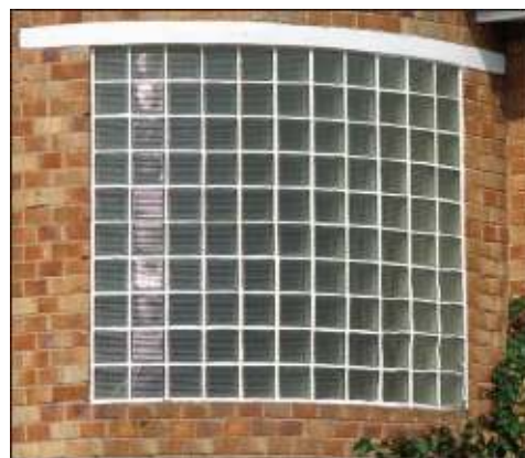
FIG 2.8: Glass bricks were introduced into the most modern houses.
