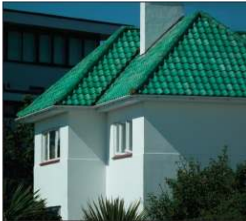
FIG 2.4: Hollywood Moderne style houses were inspired by homes from the west coast of America with distinctive green glazed roof tiles often on top of a conventional symmetrical planned structure and the odd palm tree to complete the effect.
