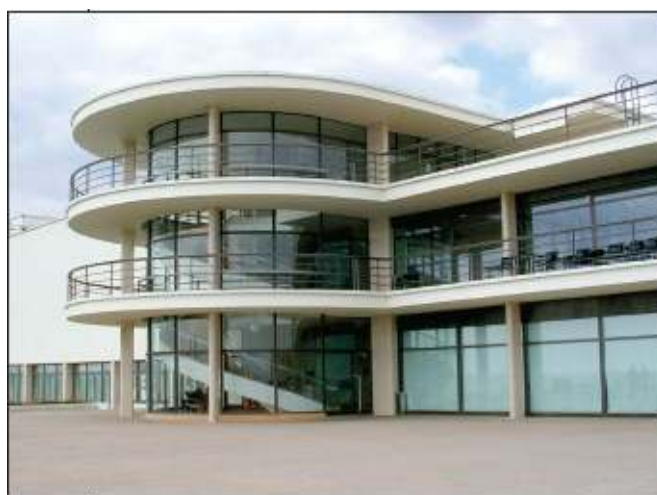
FIG 1.9: THE DE LA WARR PAVILION, BEXHILLON-SEA, SUSSEX: It was in seaside resorts that the plain, white streamlined curves of Art Deco seemed more acceptable, as with this famous Modernist pavilion designed by Erich Mendelsohn in collaboration with Serge Chermayeff in 1934.
