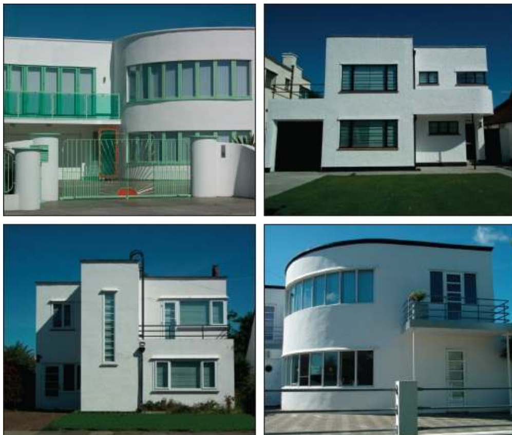
FIG 2.11: FRINTON PARK ESTATE, FRINTON, ESSEX: In 1934 the South Coast Development Company purchased 200 acres of land around Frinton, on the Essex coast, and employed the young architect Oliver Hill to design a housing estate featuring avant-garde designs, large windows and flat roofs for sunbathing. He invited designs from the leading architects working in the International Style, including Wells Coates, Frederick Gibberd, F.R.S. Yorke, and Amyas Connell, to design sections of the scheme and work commenced on around 35 houses designed by Hill and local architects close to the sea. However, the buildings were clearly too daring for local tastes and by 1935 the company was nearly bankrupt and Hill resigned the post, leaving Frinton Park Estate today as a small but rare experiment in Modernist housing.
