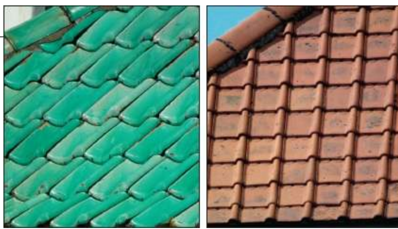
FIG 2.9: Green pantiles (left) and Roman tiles (right) are distinctive of inter-war housing, although smaller clay tiles were still the most common form of roofing tile.
