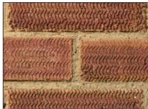
FIG 2.6: Bricks with a wavy pattern pressed into their surface were a distinctive feature of 1930s' houses that remained popular into the 1950s.
