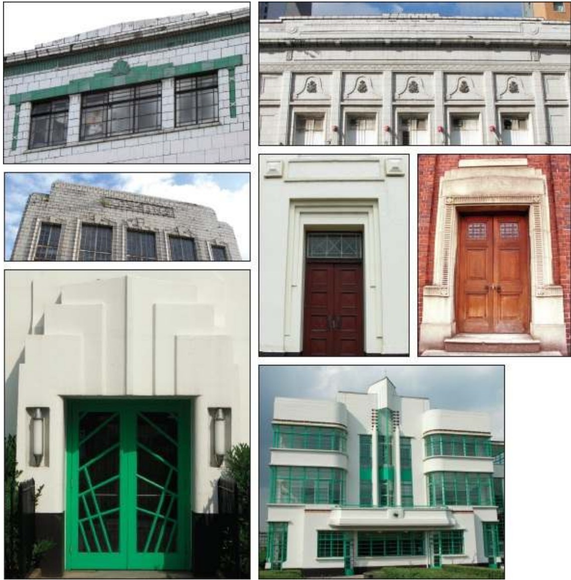
FIG 1.10: Art Deco is most notably displayed on commercial buildings, cinemas and shops where its modern form suited certain companies' profiles. Early examples have stepped profiles to the top of the building, white exteriors usually made up of glazed tiles (top examples), monumental doorways (centre right) and stylised Egyptian or Classical details. By the 1930s, exteriors are less decorative and had streamlined curves and angled steel windows. The most notable example, however, is the Hoover Building along the A40 in West London, which displays all the finest Jazz and Streamline Moderne features (bottom left and right).
