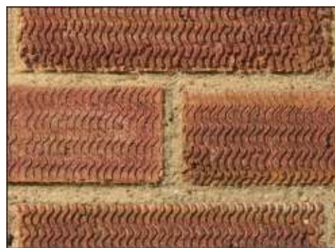
FIG 2.6: Bricks with a wavy pattern pressed into their surface were a distinctive feature of 1930s' houses that remained popular into the 1950s.
