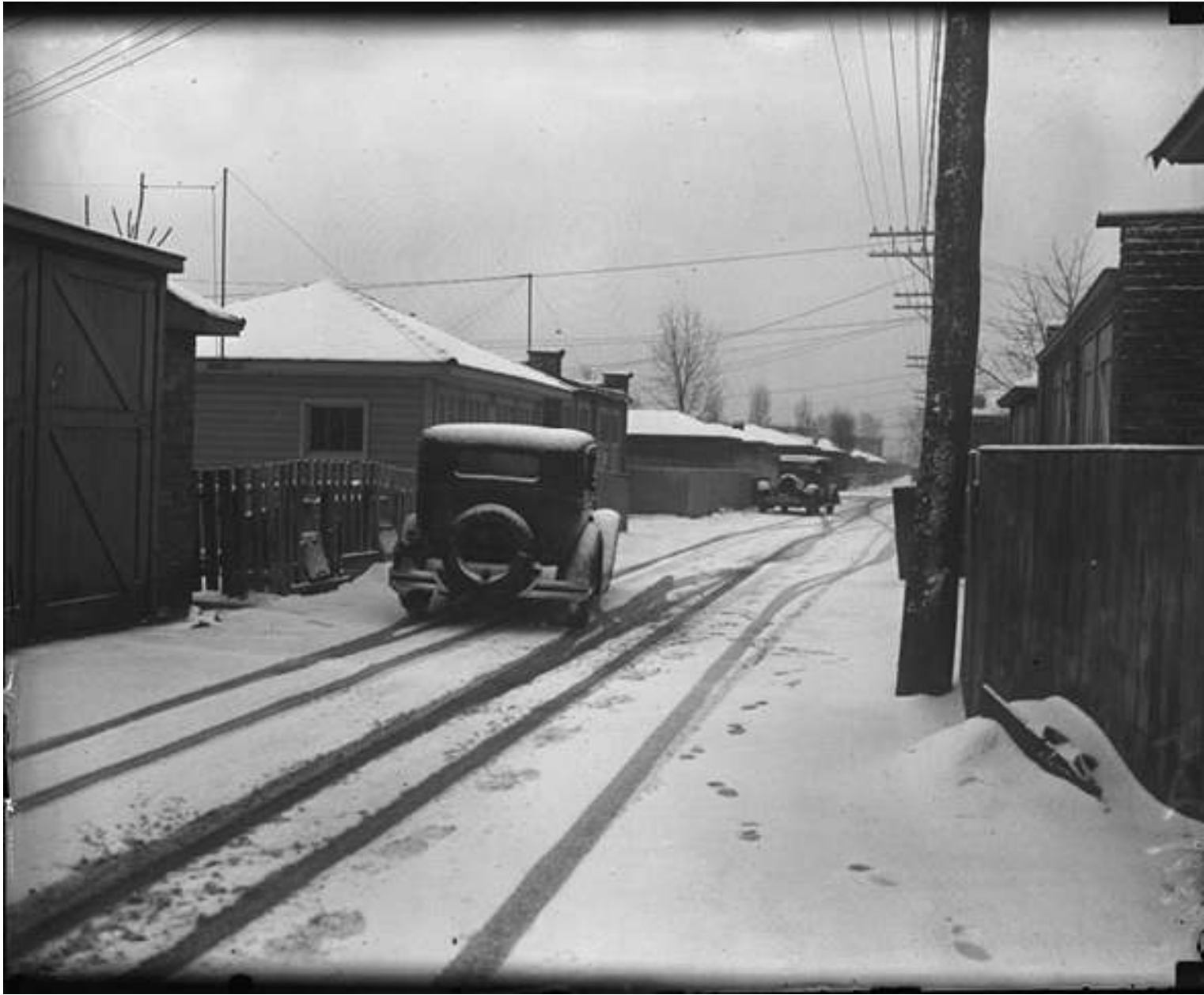
March 24, 1930: The alley behind Al Capone's home.
