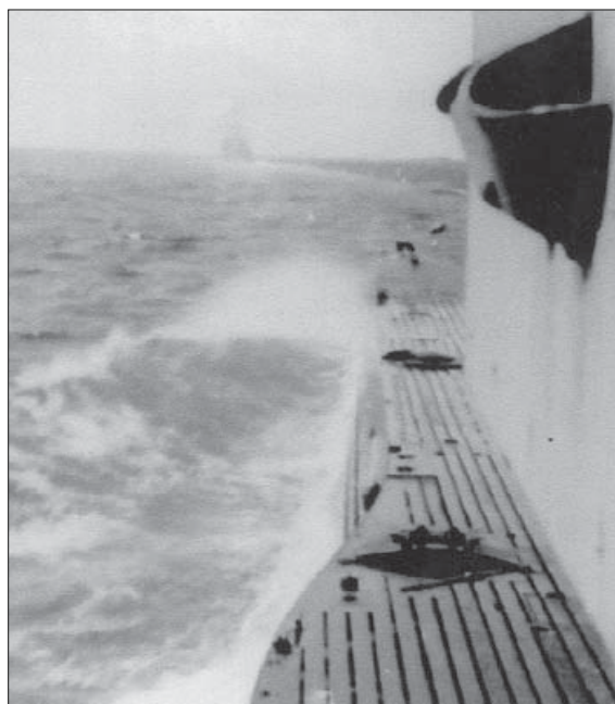
BELOW A Type VIIC on training exercises in the Baltic. Note how narrow is the width of deck available for passing along the side of the tower. The Type IX was, by comparison, far more spacious.
