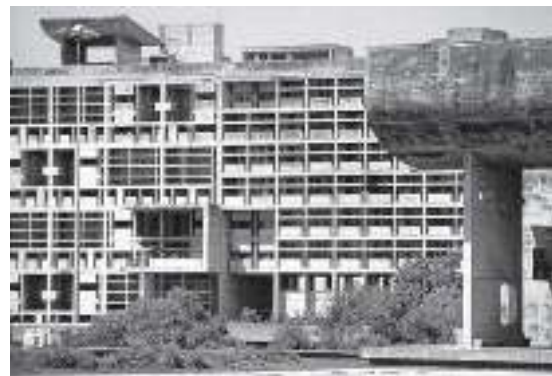
Chandigarh, parliament chamber — Chandigarh, administrative offices
