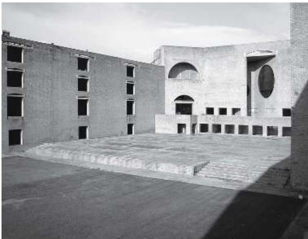
IIM courtyard complex with library — Kanchanjunga apartment building
