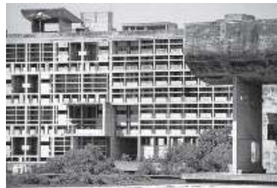
Chandigarh, parliament chamber — Chandigarh, administrative offices
