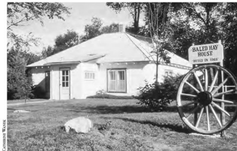
1-3: The Martin/Monhart home, built in Arthur, Nebraska in 1925, demonstrates the elegant simplicity and endurance of straw bale construction.
