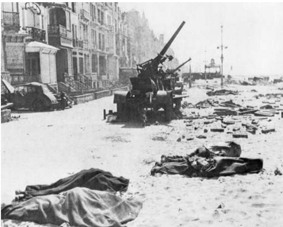
7 Devastation at Dunkirk. Nevertheless, the bulk of the BEF escaped capture.
