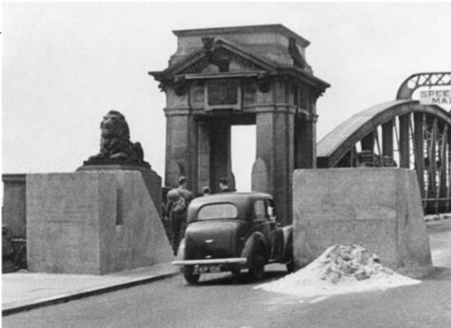
12 Concrete blocks at a bridge on the GHQ Line.
